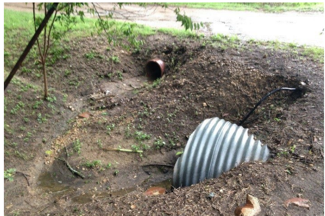
Figure 6E: Undamaged Culvert Example
