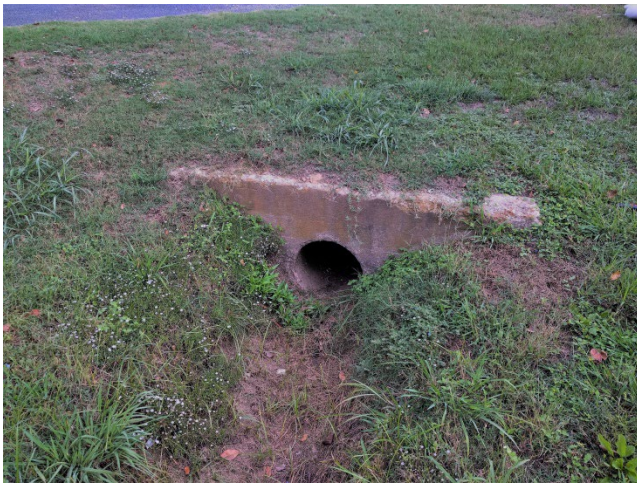
Figure 6A: Roadside Ditch & Concrete Culvert Example
