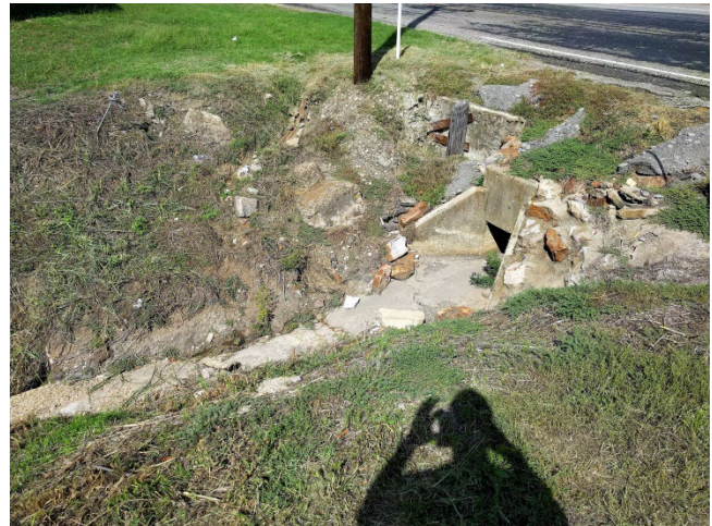
Figure 6B: Roadside Ditch Example
