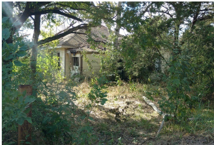
Figure 3B: Overgrown Yard/Dilapidated Housing Example
